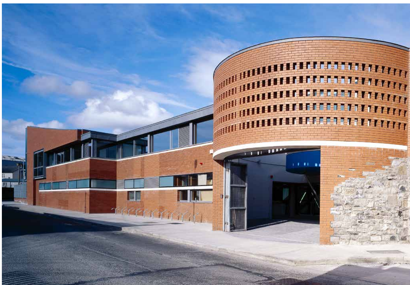
Foyer Housing and Training, Dublin
