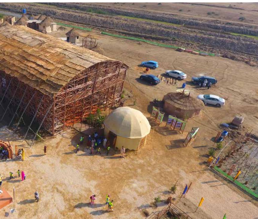
Bamboo and earthen community centre, Makli, Pakistan
