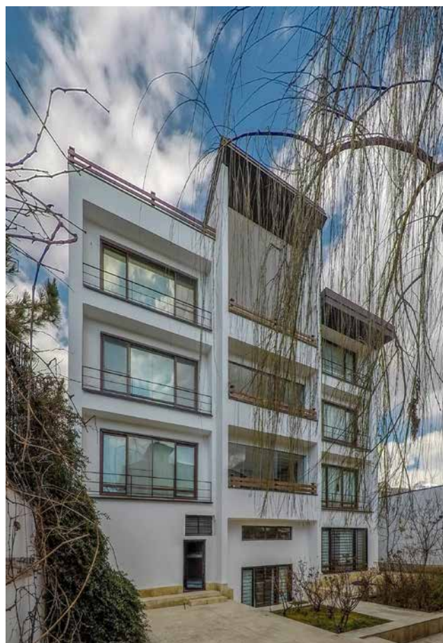
Apartment No.20, Lavasan, credit: BonnArq Architects Principal Architect: Parshia Qaregozloo
