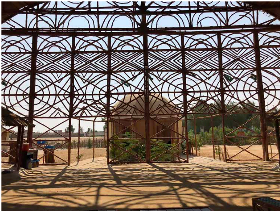
Zero Carbon Cultural Centre - View of Entrance from inside
